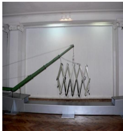
Unfolding single-span reusable bridge ( L = 48 m)
