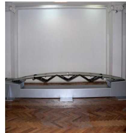
Unfolding single-span reusable bridge ( L = 48 m)
